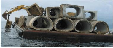
On October 14, a Barge Load of Culverts was deployed in FH-1 near Barge B. The surrounding depth was 64 feet, the tide was 1.5 feet, winds were from the East at 12 knots.
